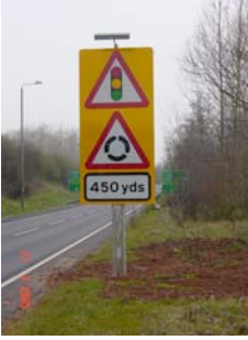
Typical Illuminated Sign on Lattix Mast
